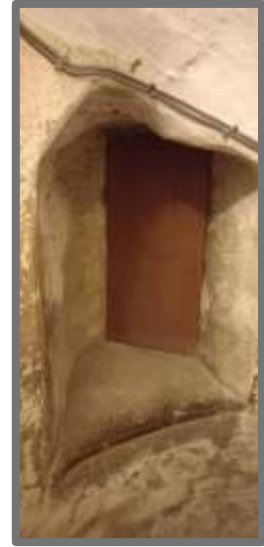
Access to former rood-loft, from stairs to bell tower.
