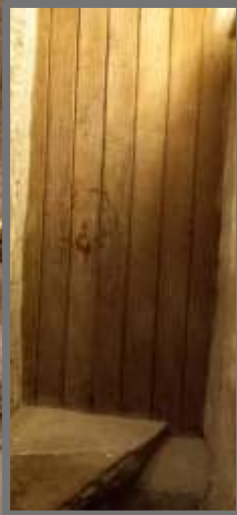
Interior of door accessed via stairs to bell tower.
