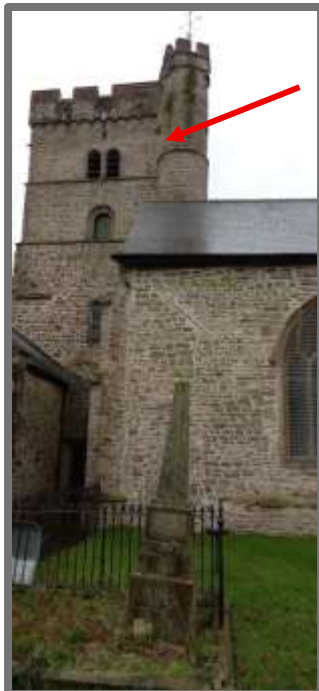
External view of the angle/stair turret.
